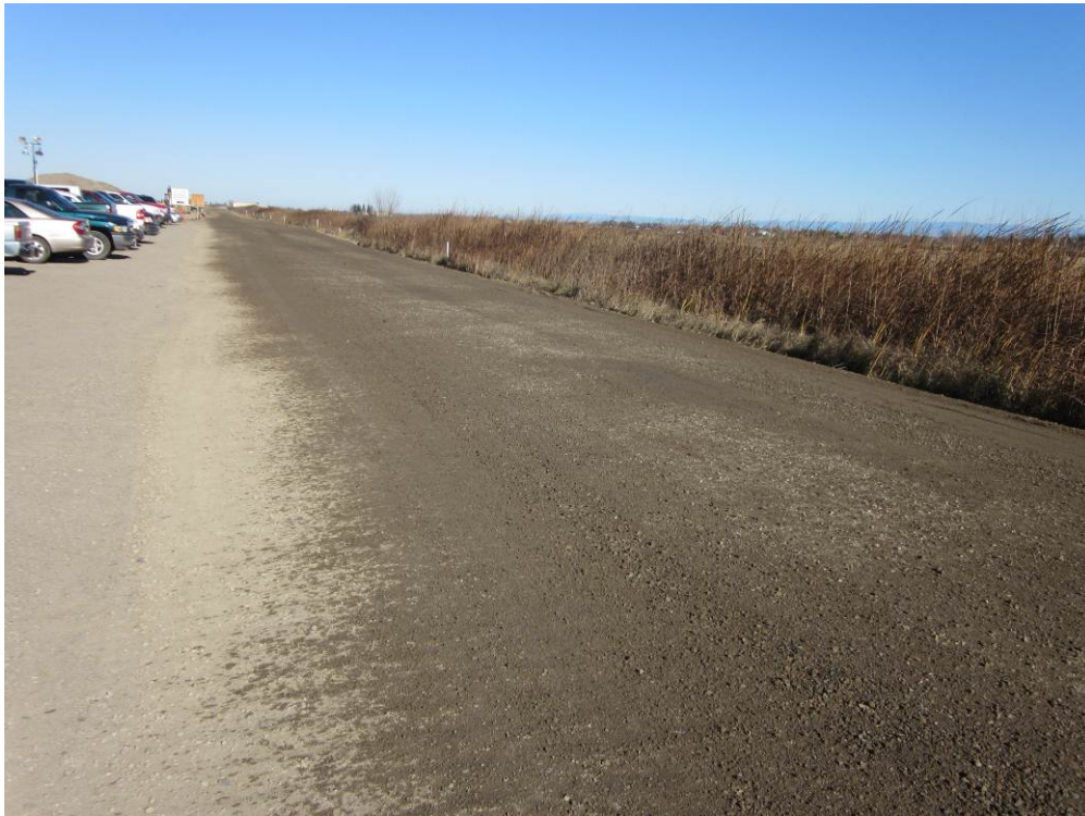
Photo 2: McAusland Road adjacent to the Compressor Station site immediately following water application for dust control.
