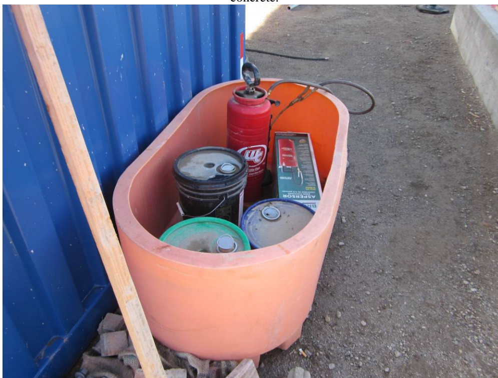
Photo 4: Liquid hazardous materials storage at the Compressor Station site observed to have adequate secondary containment.
